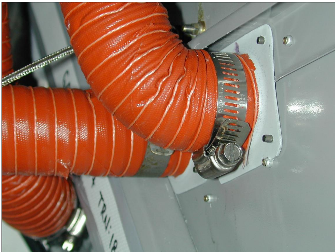
Figure 3: Completed RHS modification viewed from inside the aircraft.
