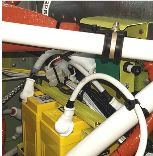
Figure 2: Installed batteries (GA8-TC 320)
