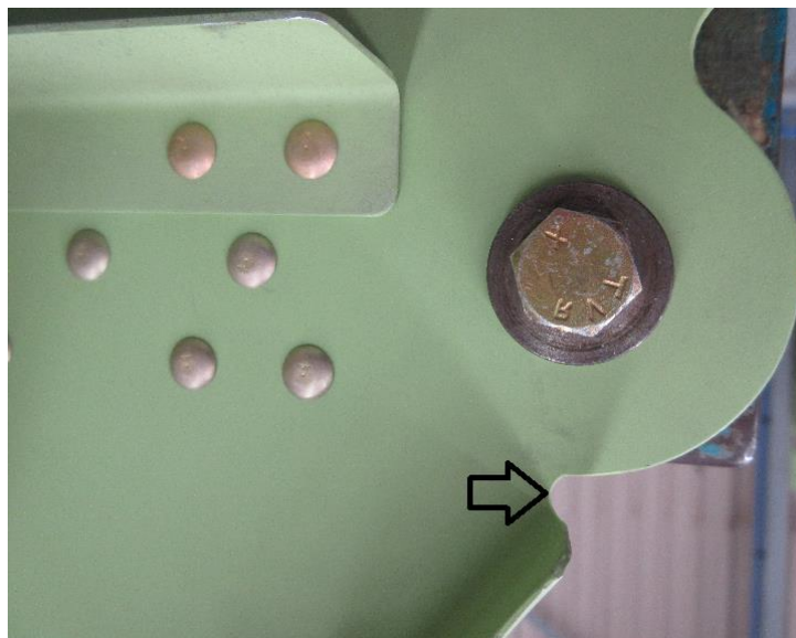
Figure 4: Area of Rib for Inspection
